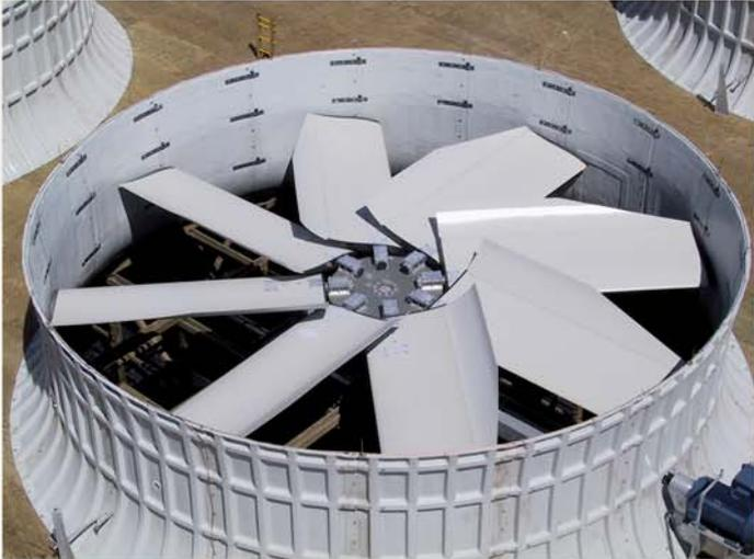
32' 60F Fan installed in CT
